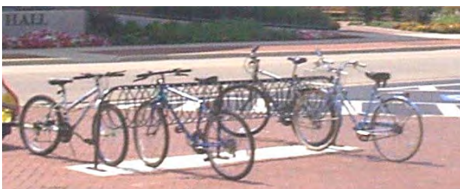
JH5 suspended helical loop (straight end verticals): Westmont Station ( note: more loops per foot )
