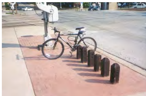
PW wooden post (difficult to place locks in holes, thus these racks are rather unusable)
