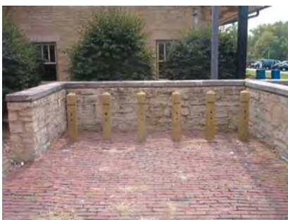
PW wooden post (difficult to place locks in holes, thus these racks are rather unusable)
